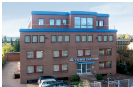
Another storey added to TEWS Elektronik building in Hamburg, summer 2005
